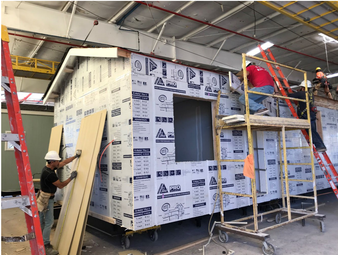
Figure 5: Installation of foam sheathing at plant. EPRI. 2022
