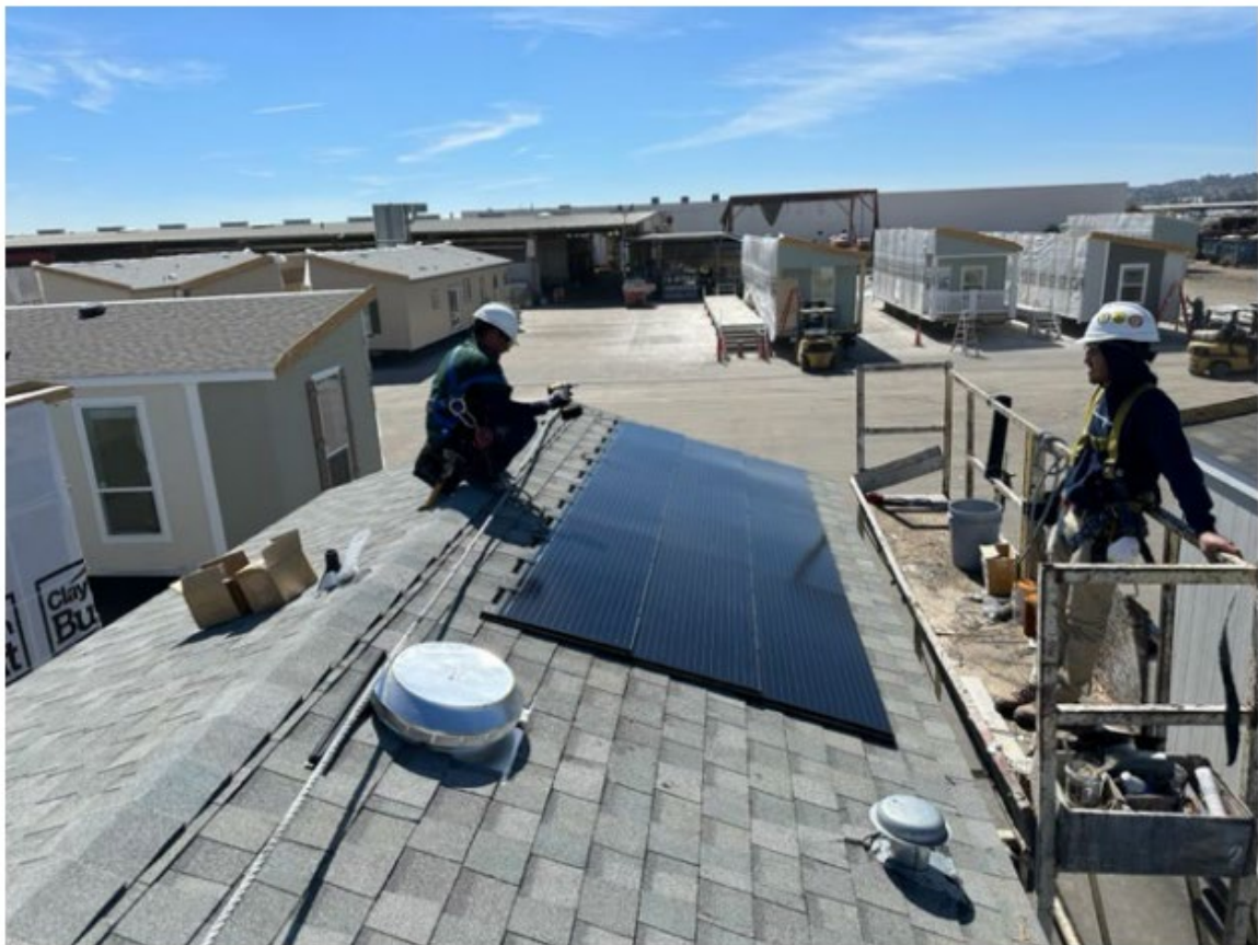
Figure 2: Solar PV shingle installation in plant yard. EPRI. 2022.
